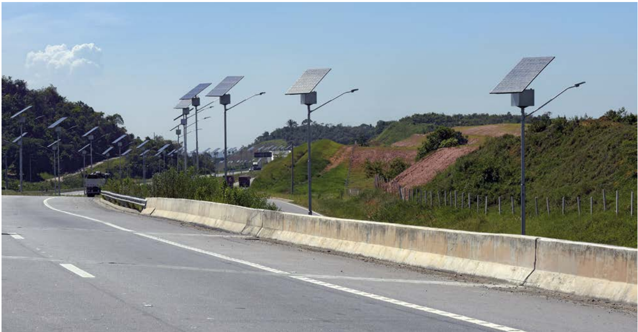
Solar panels used for street lighting in the Metropolitan Ring of Rio de Janeiro
